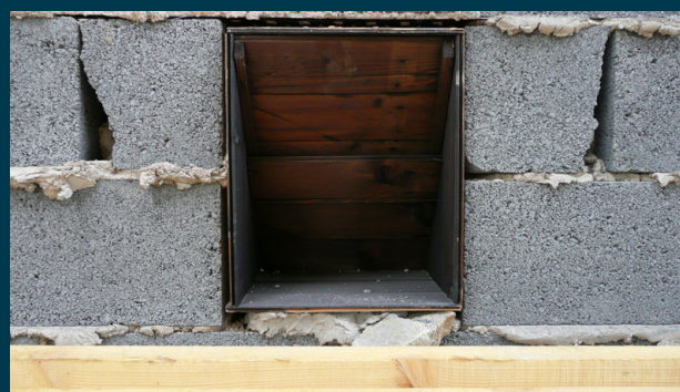
Hopper providing sheltered fly-in access (see Schofield, 2008).
