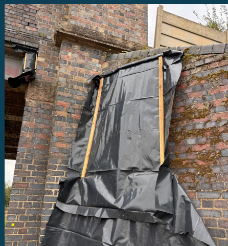
Inset 7: Exclusion device in place
