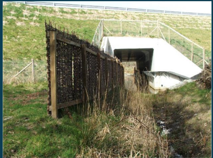
Culvert with hurdle fencing guide
