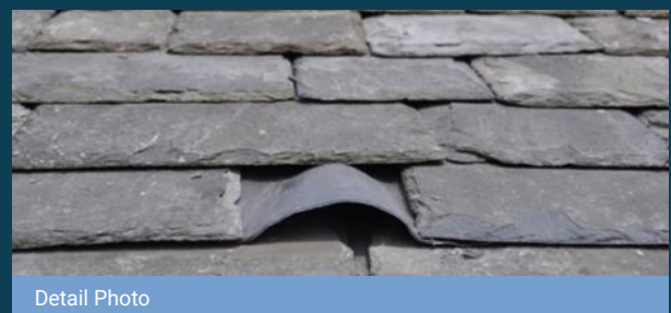
Bat access point at gable apex
