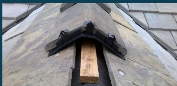
Ridge tiles showing tile and plastic union installed over batten
