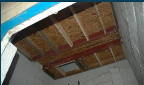
Internal – ceiling inserted 1.5 m below flat roof
