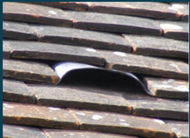
Bat slate in position (neat and unobtrusive).
