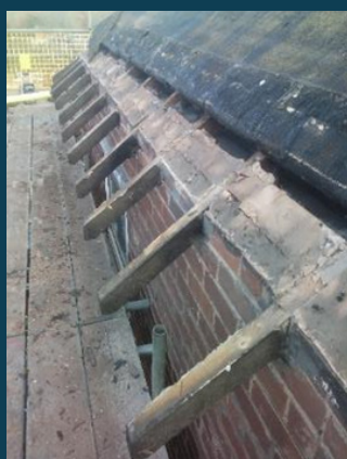
Stripped wall plate
