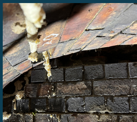
Inset 4: Previous Myotis roost deconstructed by removal, prior to filling with expanding foam
