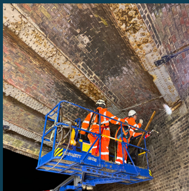
Inset 5: MEWP used to facilitate endoscopic survey
