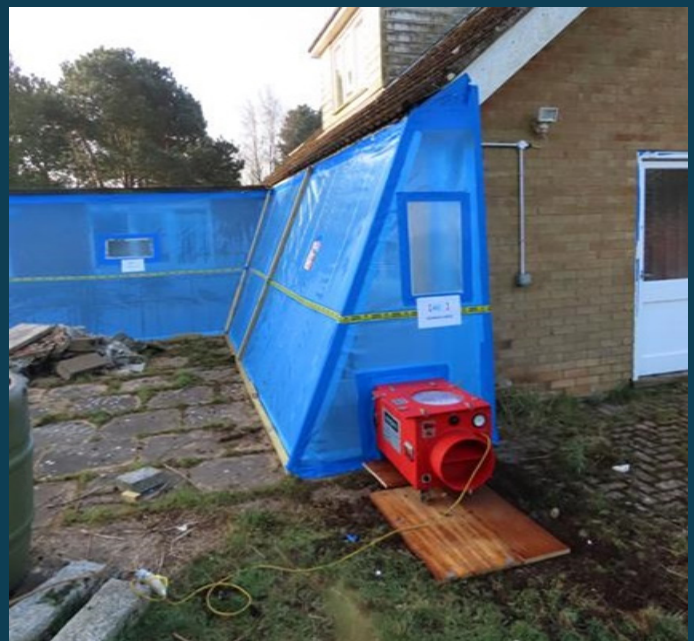
Negative Pressure extractor pump and filter
