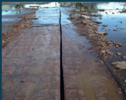
Diamond cut through culvert slab
