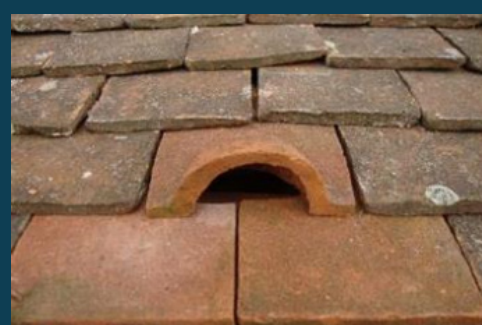
Bat access tile installed within the farmhouse roof
