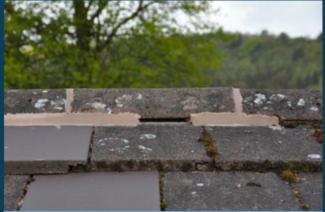
Ridge access, wet ridge (P. Waring)
