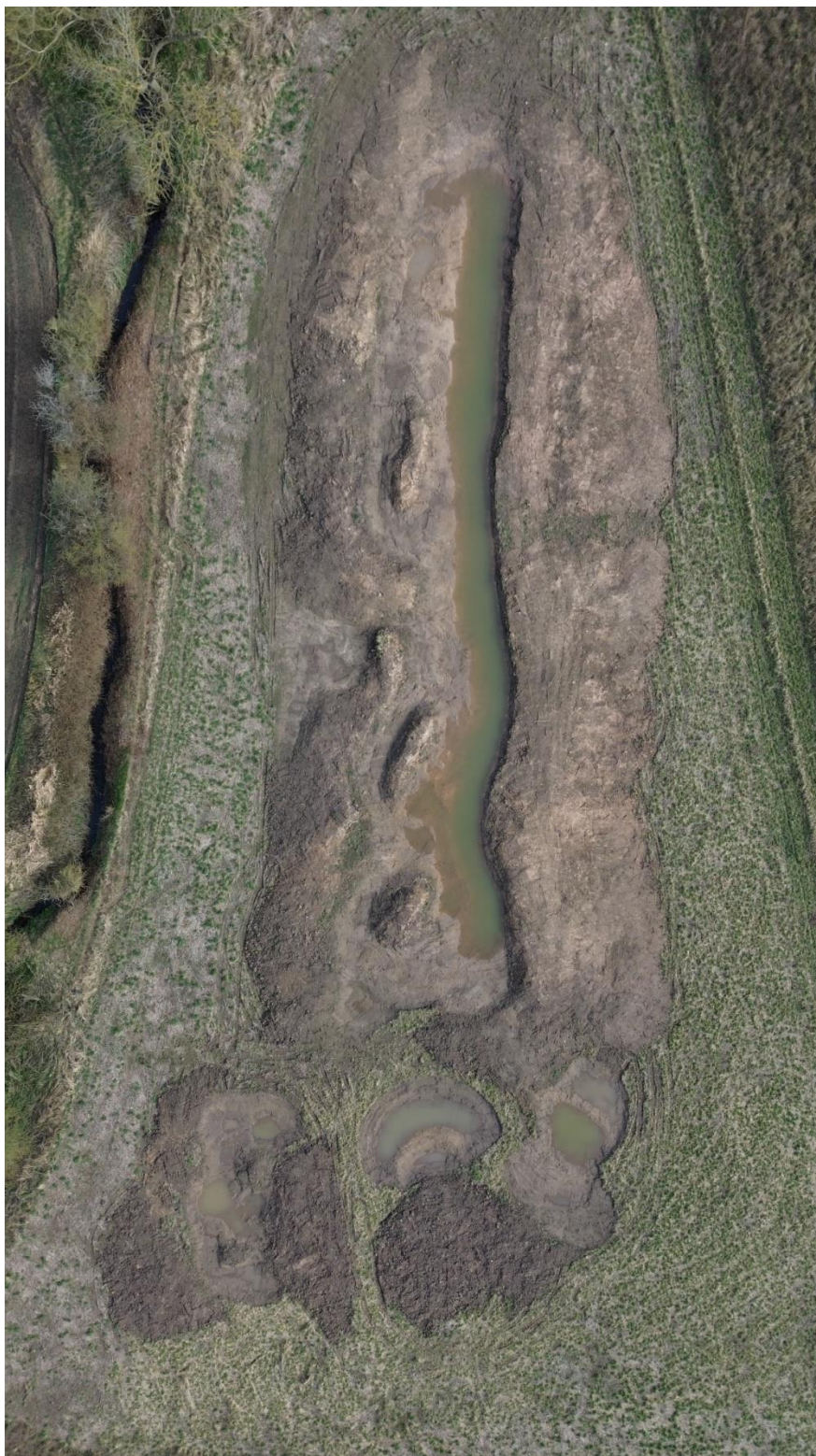
Wet underused field corner after capital works – wetland and meadow creation (credit Andrew Wolfenden)
